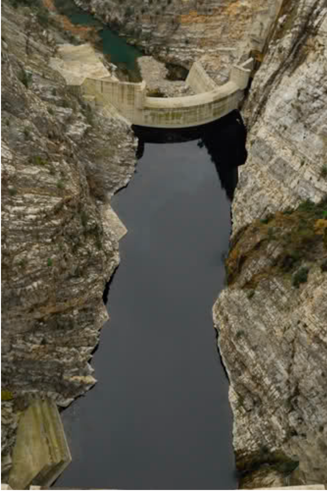
Berke Barajı; Ceyhan
