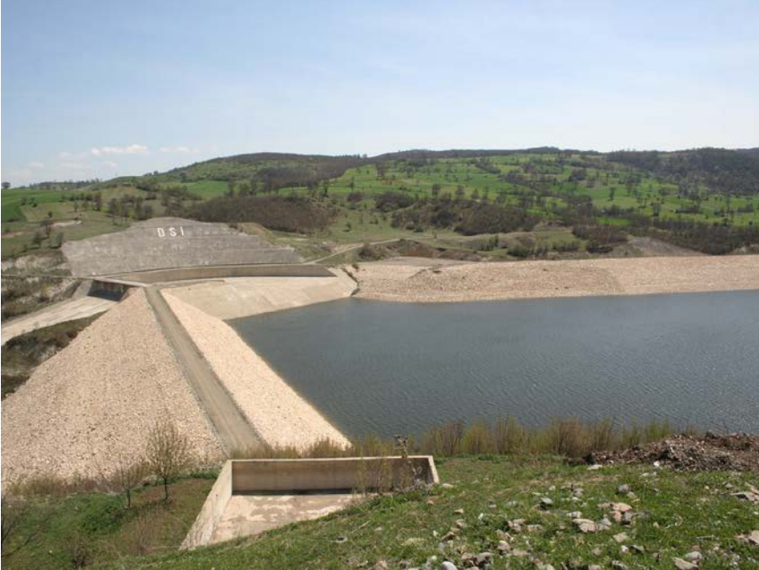
Toprak dolgu baraj
