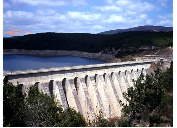
Beton payandalı baraj
