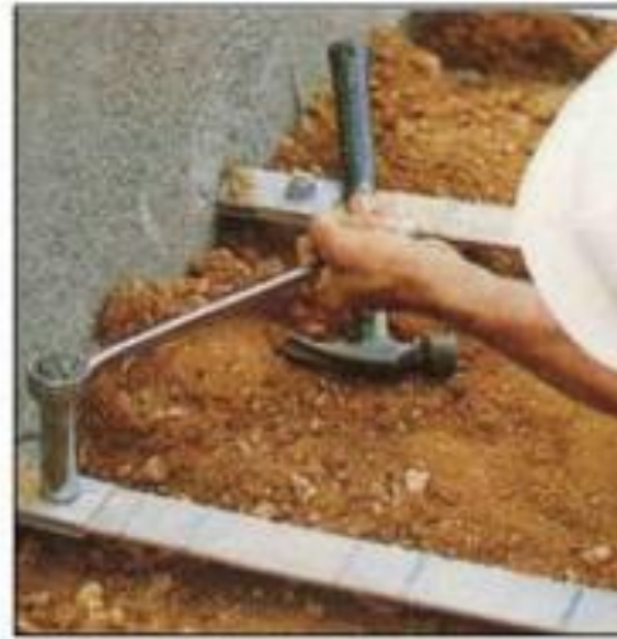
Attaching strip reinforcement to the facing panel
