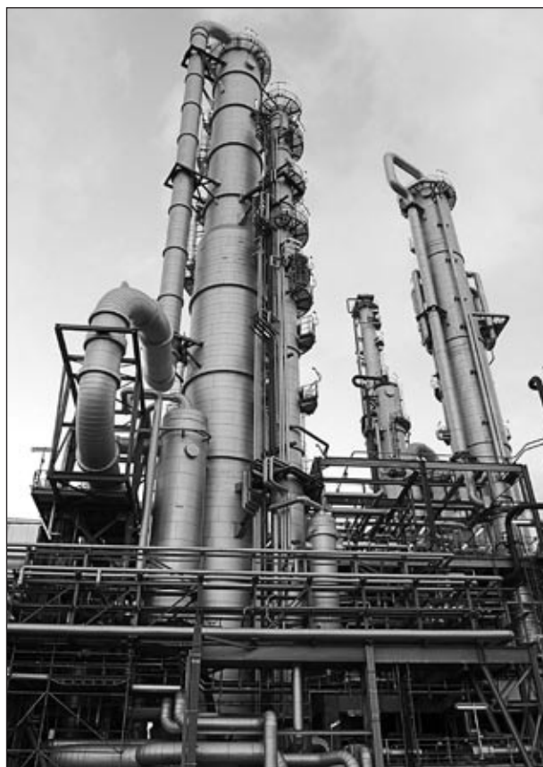
FIGURE 1 The new HPPO plant at the BASF site in Antwerp, Belgium, completed the startup phase in 2009. With a new process for producing propylene oxide jointly developed by BASF and Dow, wastewater is reduced by up to 80 percent, and energy use is reduced by 35 percent compared to conventional processes. Source: BASF.
